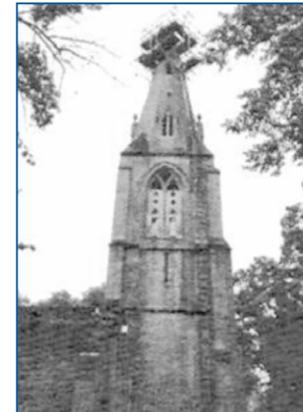
Mary's Bainton Spire Repairs
