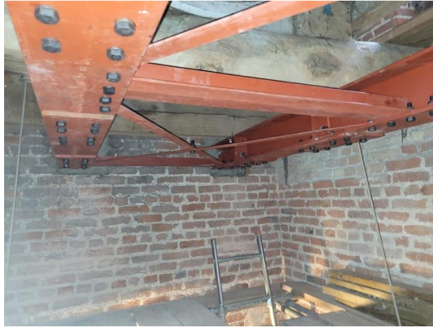
New steel beams in situ in the belfry. 2 nd November 2023
