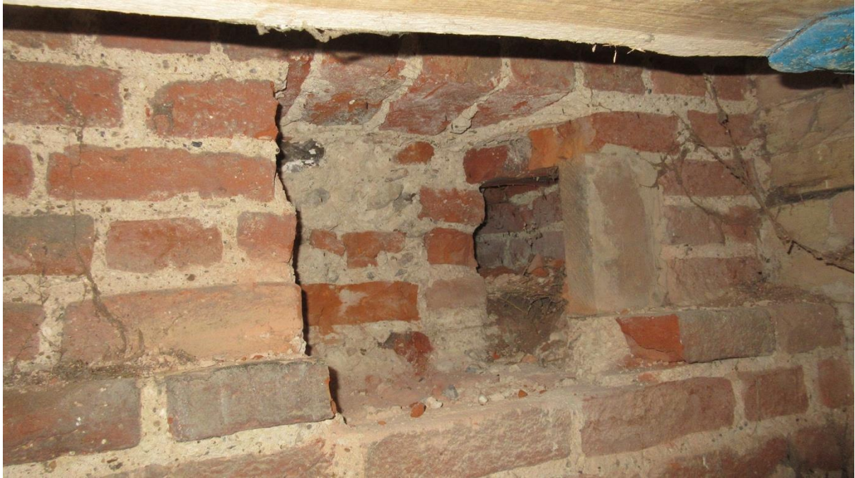
Cracks in the interior belfry masonry walls.
