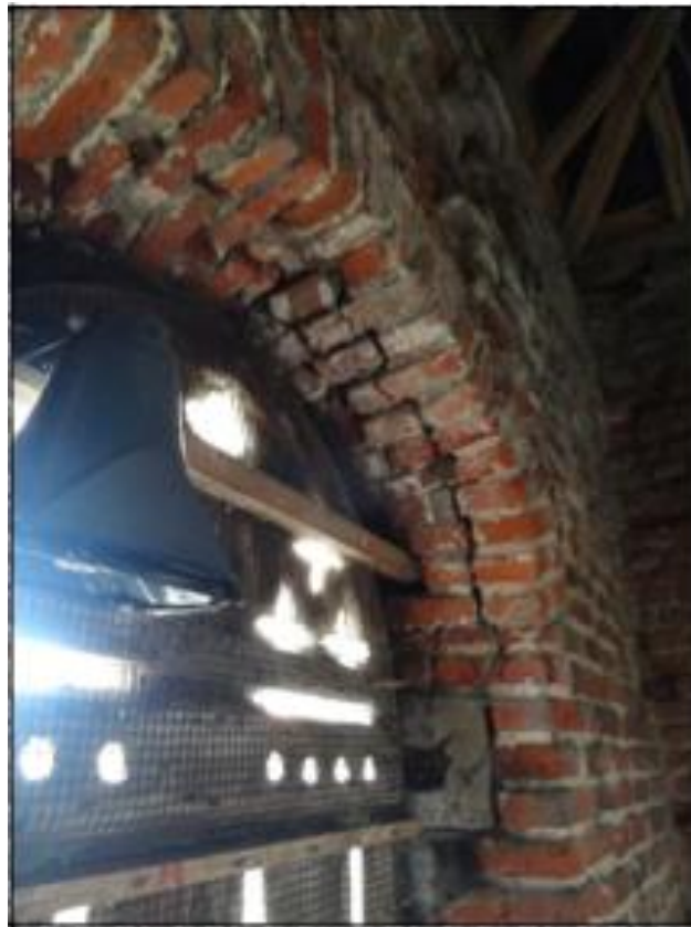
Cracks around belfry opening east prior to works commencing.
