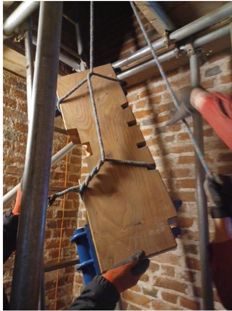
Lifting the headstock up into the belfry.
