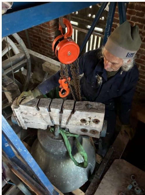
November 24 th 2023 removing the old tenor headstock
