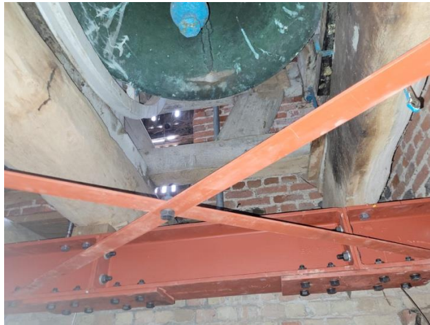
New steel beams in situ 2 nd November 2023.
