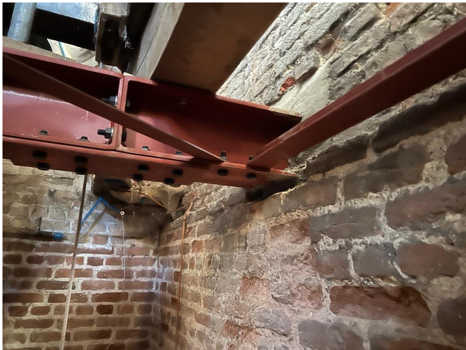
New steel beams 1 st December 2023
