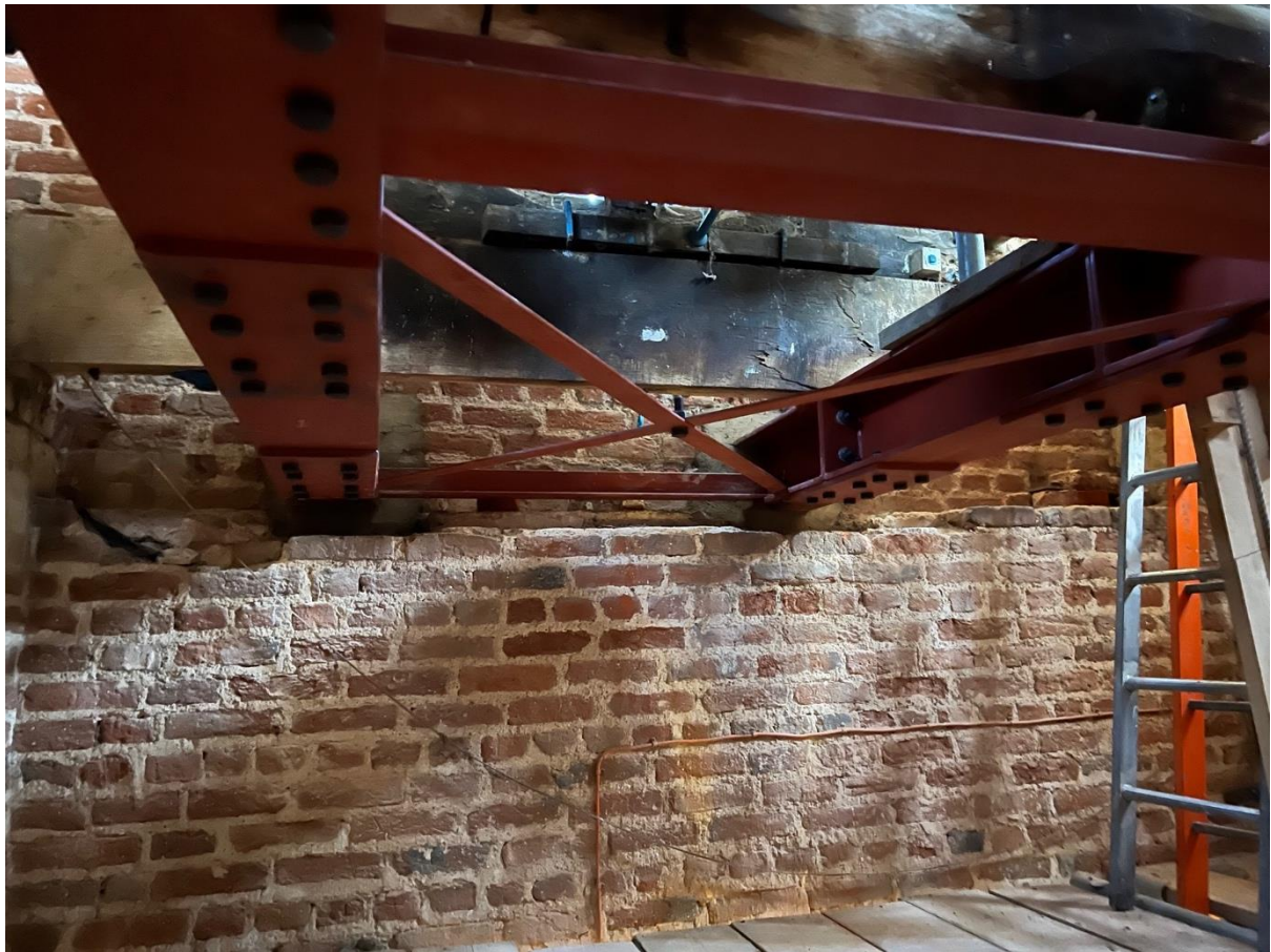
New steel beams 1 st December 2023
