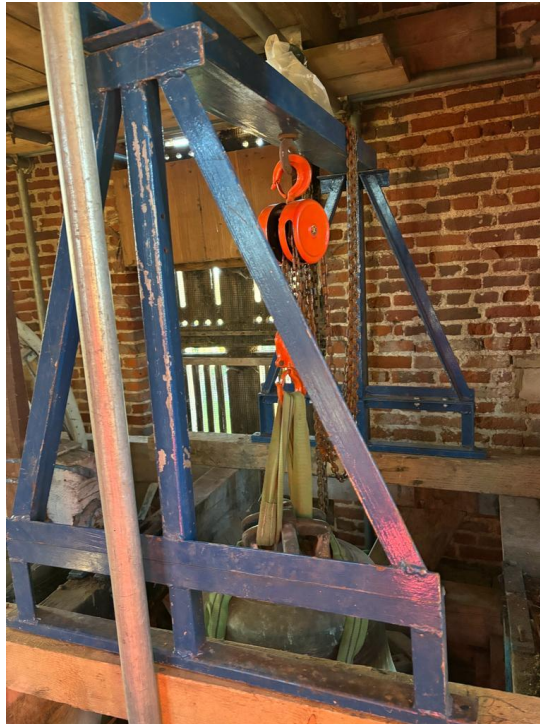
Securing the 4 th bell without its headstock.
