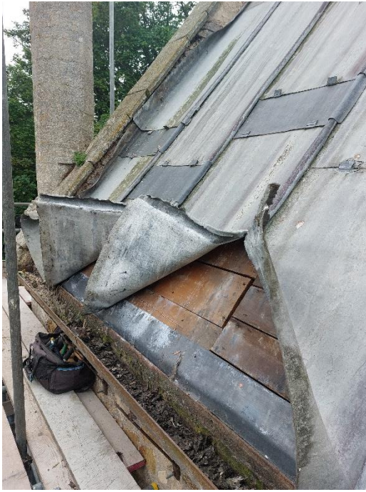
Plate 1 Failing lead was removed
