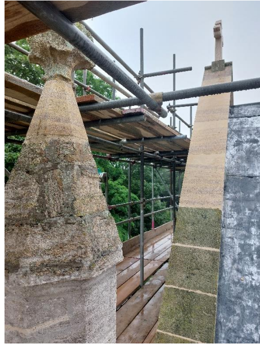
Plate 2 Apex stones were replaced
