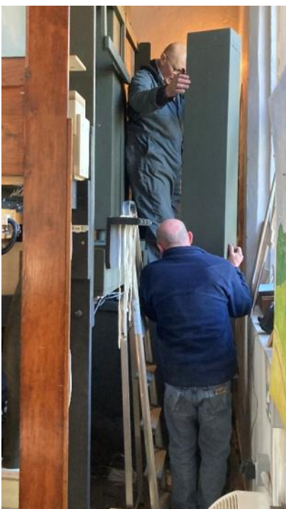
18 th March: fitting the Pedal Bourdon pipes
