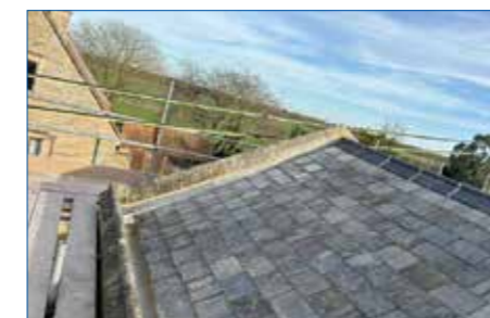
Etton, St Stephen, Chancel Roof completed in 2026.
