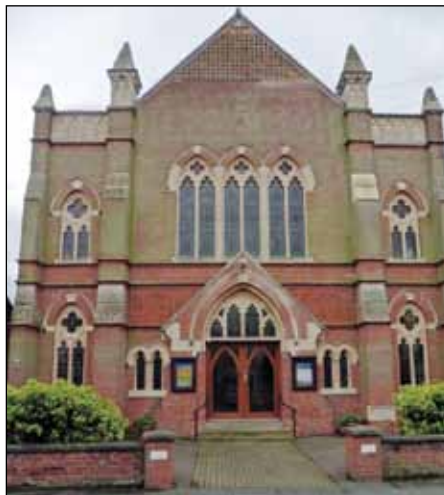
• Ely Methodist Church. The Trust gave a grant of £1000 towards the renovation of this facade facing Chapel Street.
