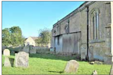
All Saints, Elton – The old boiler house soon to be replaced?
