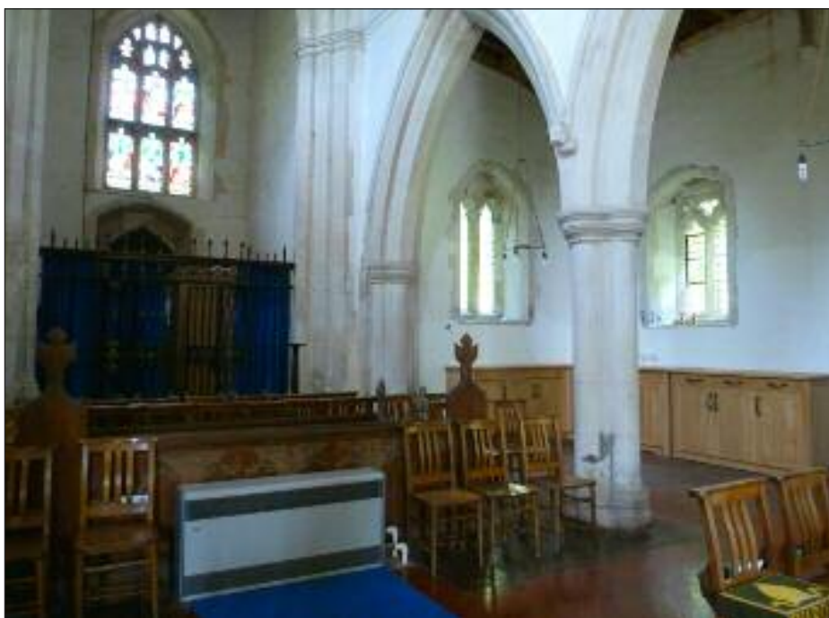
• We contributed a £3000 grant and £15,000 loan to a £70,000 scheme to install a toilet pod in the base of the tower with a servery and storage around the west end of the north aisle.
