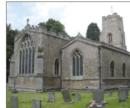
• Holy Trinity, Orton Longueville. The Trust offered a loan of £20,000 and a grant of £5,000 towards an extension for new facilities being added to the north of this Grade 1 church.
