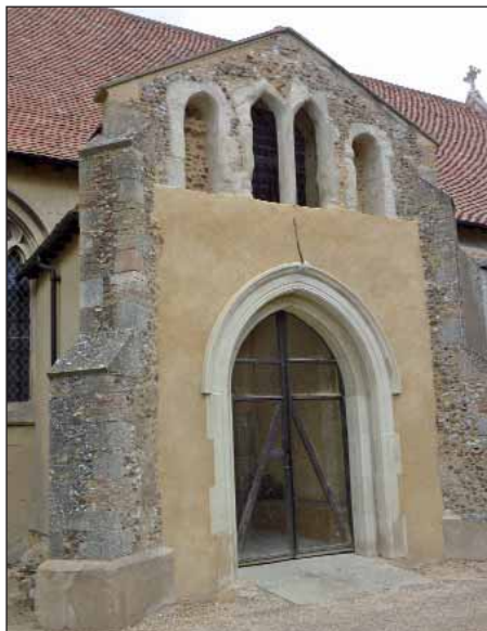
• The repaired south porch front at Barton; £3000 WREN grant, £4500 CHCT loan
