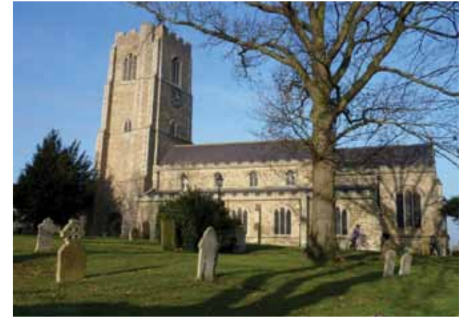
• St George Littleport, offered a loan of £15,000 towards tower repairs.
