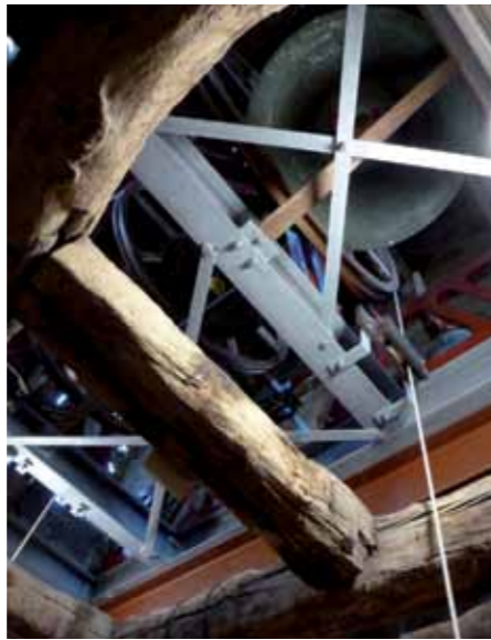
• The new frame
