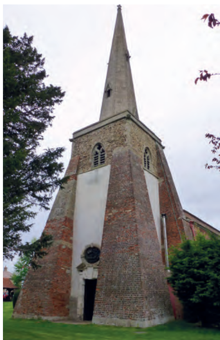
• The well buttressed west tower of Conington St Mary, visited by the trust in May 2013.
